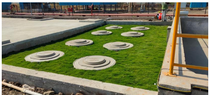
Field installation — rainwater harvesting chamber
